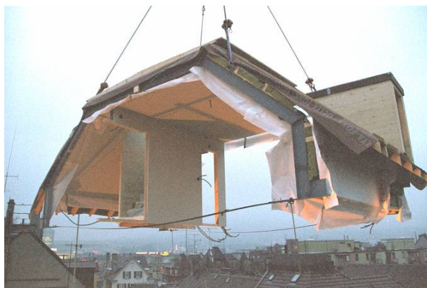
Figure 4 : Use of prefabrication for high efficiency retrofitting (IEA ECBCS annex 50) [14]
